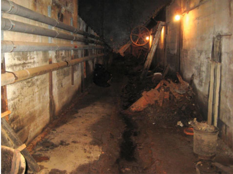
A coal ash hopper is visible suspended from the ceiling. Debris and groundwater are visible on the floor.
