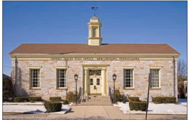
The Mercersburg Post Office (1937) is based on the Colonial revival style plan but is faced with field stone rather than the more typical brick .
